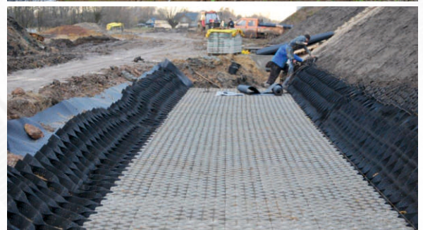
Protective channels in the geocells system. Soil-filled geocells covered with grass.
