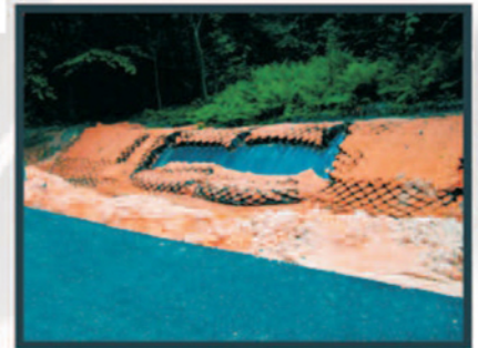
Example of flow of surface wrongly installed geogrid
